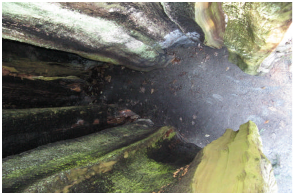
Photo 6: Looking down centre of Hollow Tree at weakened "C" shaped cross section
